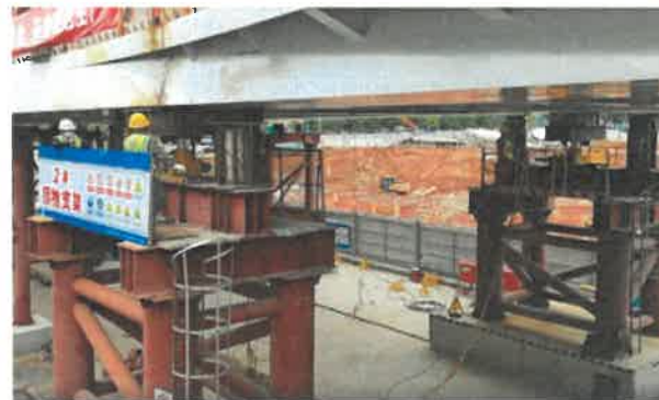
顶推施工 参考图例3-2-14
